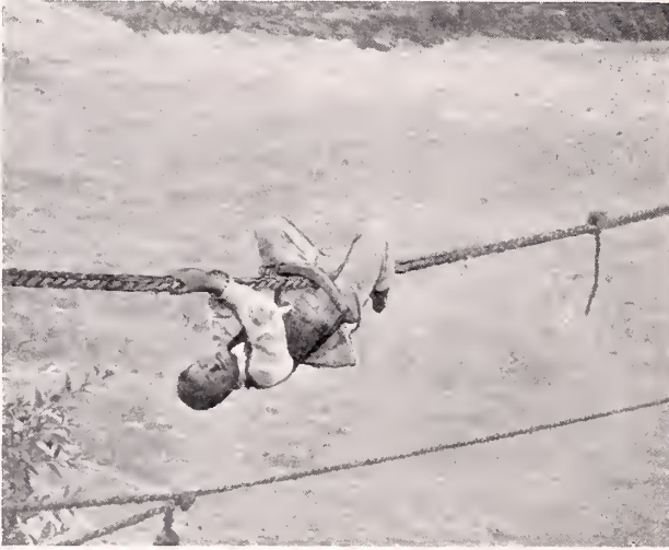
NATIVE CROSSING ROPE BRIDGE
